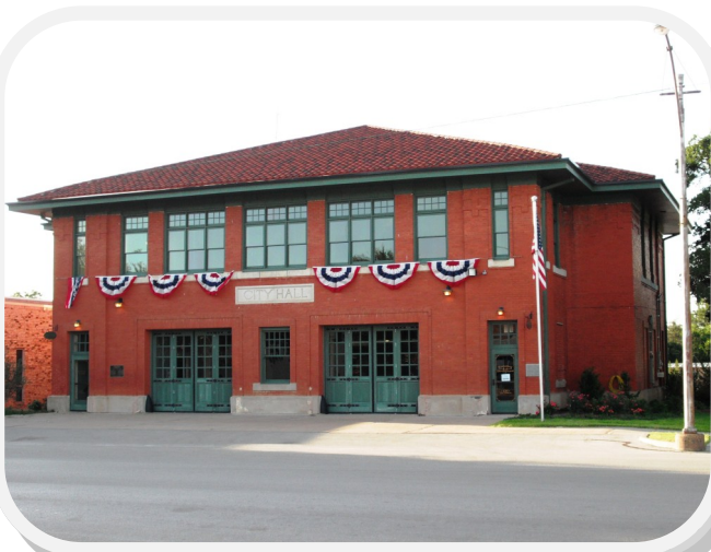
Hillsboro Historic City Hall 127 E. Franklin Street Downtown Hillsboro Texas
